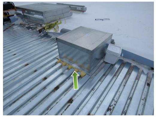
We should be making sure that our scope sheets include installing a low rise SPF in the flutes (above & below) in order to close off any air pathway.
